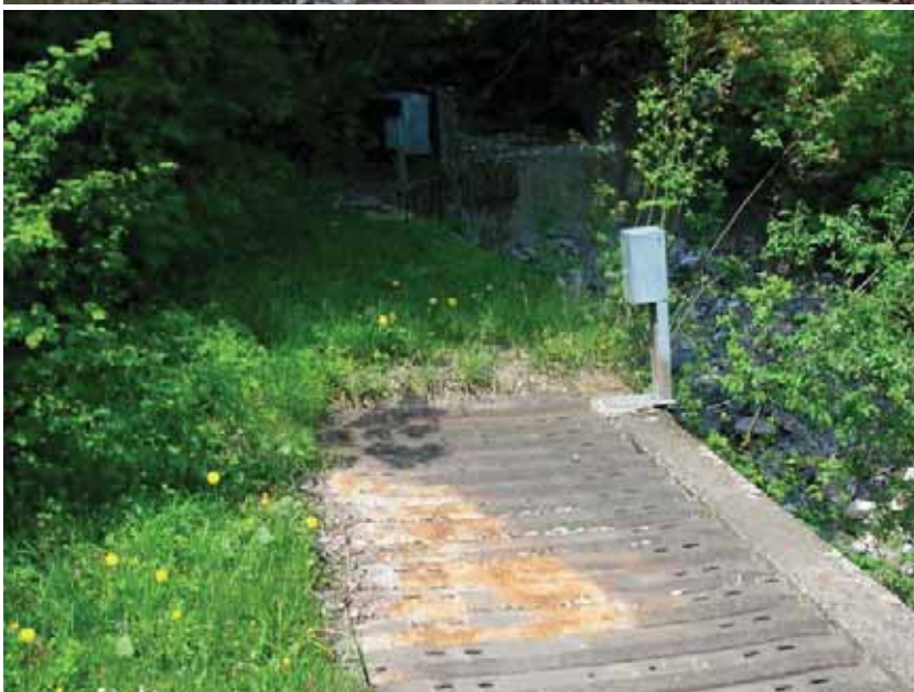
Fassung Gerbibach, Sandfang
