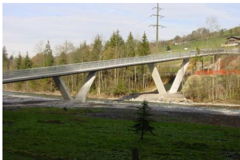
Brücke Heustrich, Emdthal BE i = 11.5\% , 1'100 m.ü.M.
